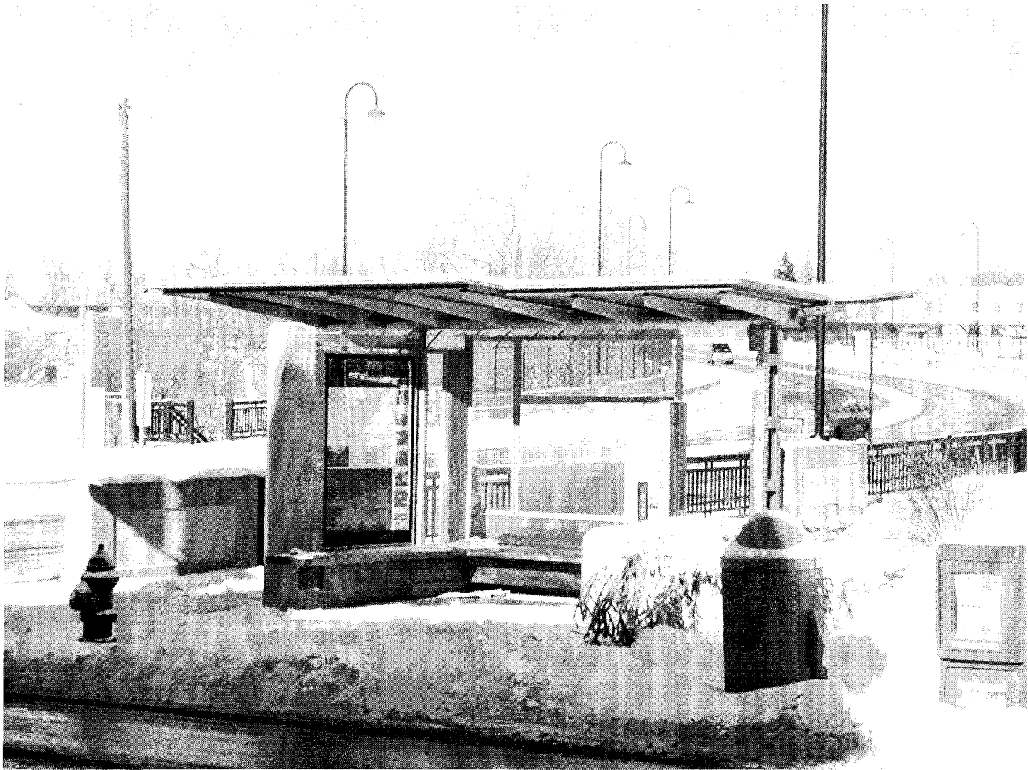
While providing protection from the elements, the Bus Shelter maintains visual connection on all sides.
