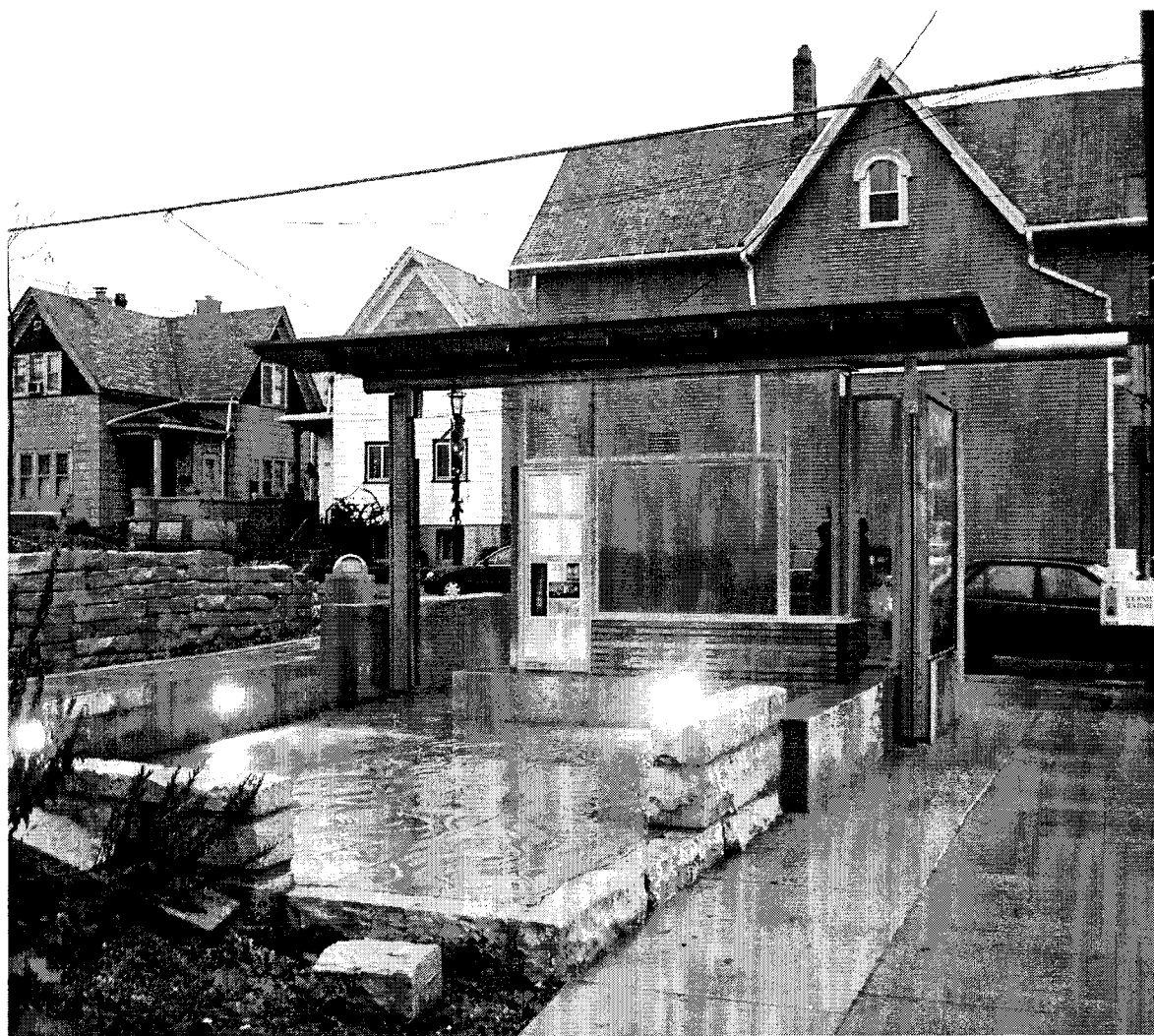
View of Shelter as approached from the Marsupial Bridge.
